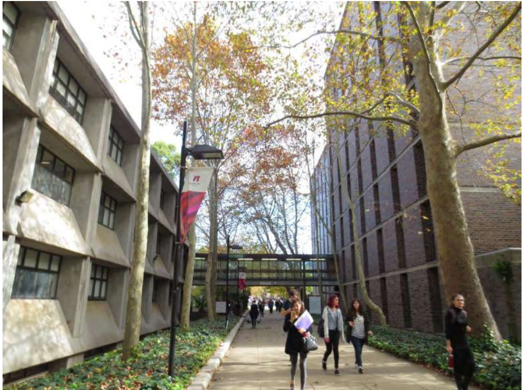
Figure 24 Plane trees adjacent to the building are stunted due to shade and proximity to the building
