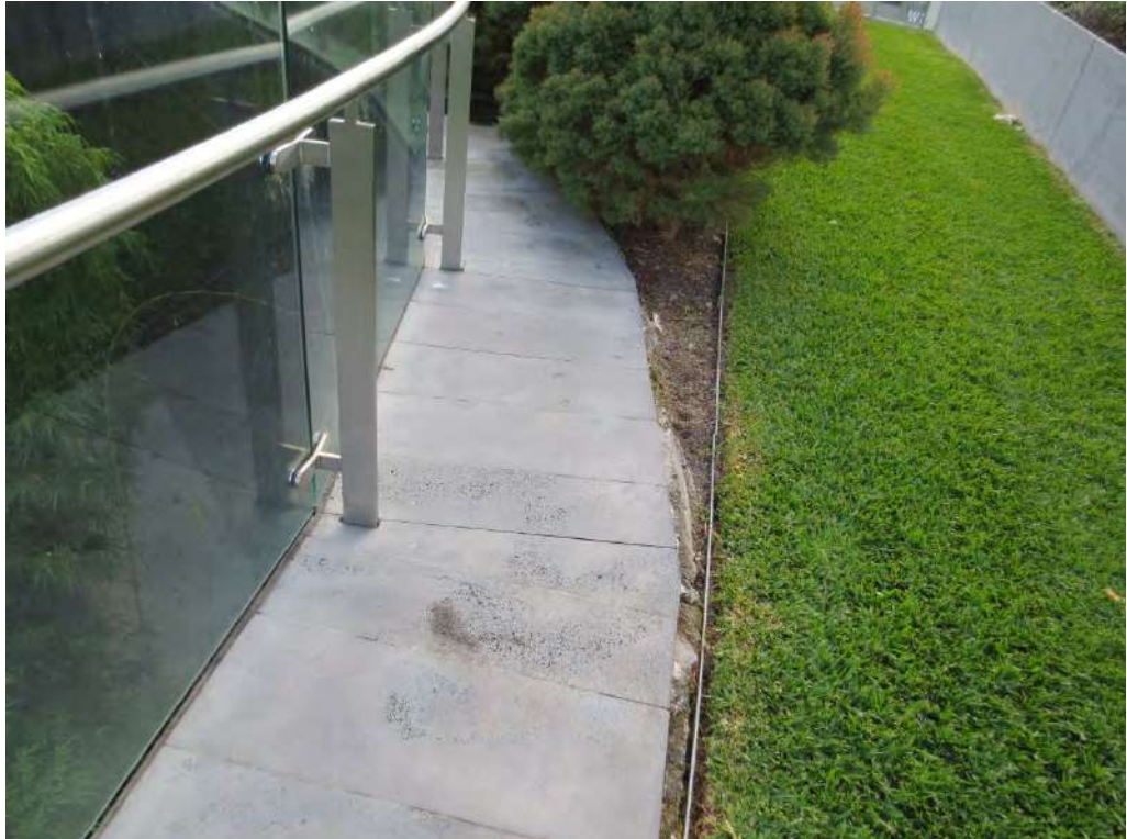
Figure 17 Planting and lawn over a concrete slab near the library. Note the shape of the garden bed results in an area too narrow and difficult to plant. A different resolution could have prevented this.
