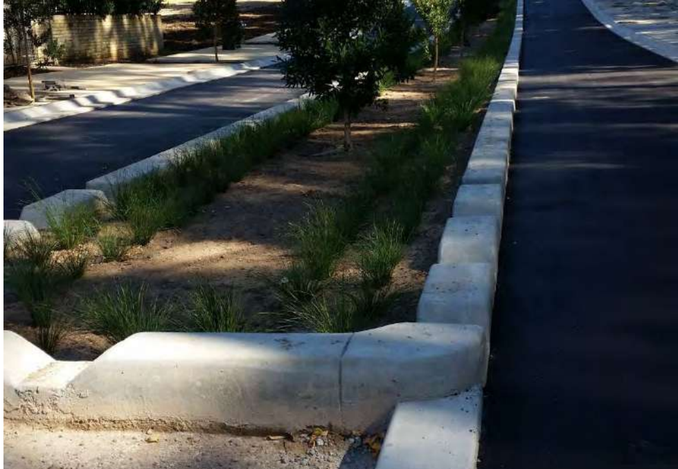
Figure 21 "Castellated kerb" allows water into the central median where it is "polished" by vegetation and slowed from entering the stormwater system. Planting benefits by being passively watered.
