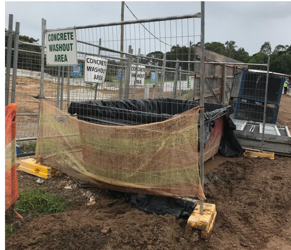
Photo 8 – Designated concrete washout area.
