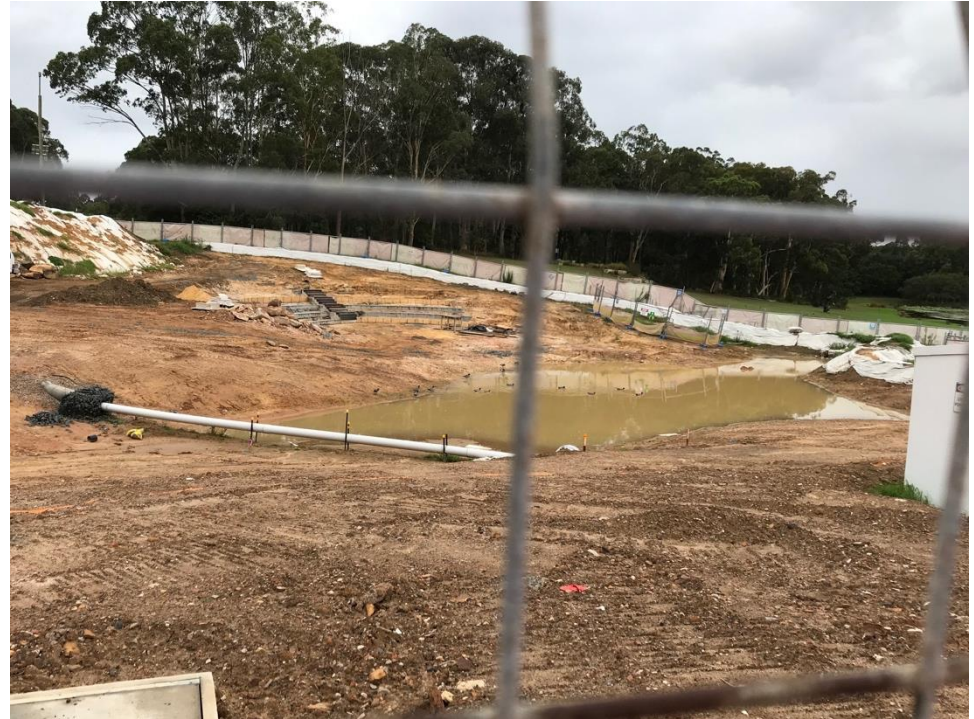
Photo 2 – Sedimentation basin in place with good capacity and controls.
