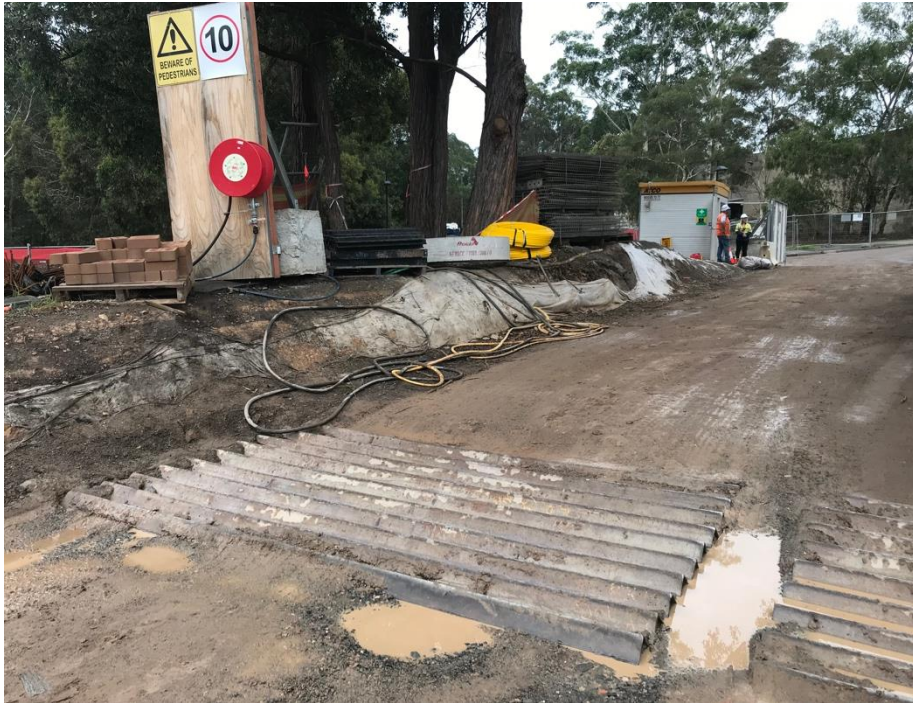
Photo 9 – Rumble grid in place at site vehicle entrance and wheel washing.
