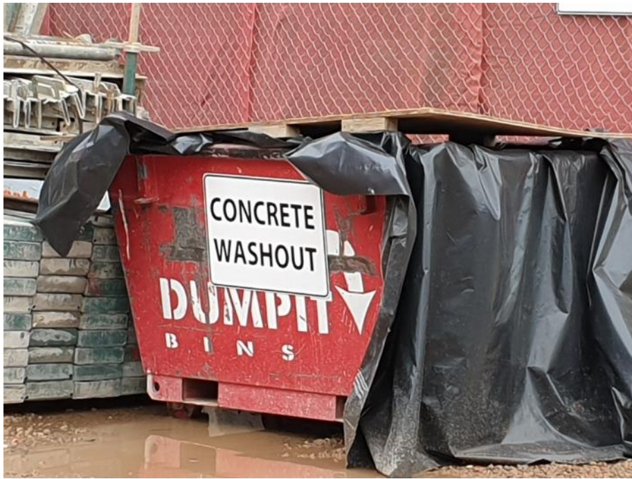
Photo 6 – Concrete washout bin available at point of use.
