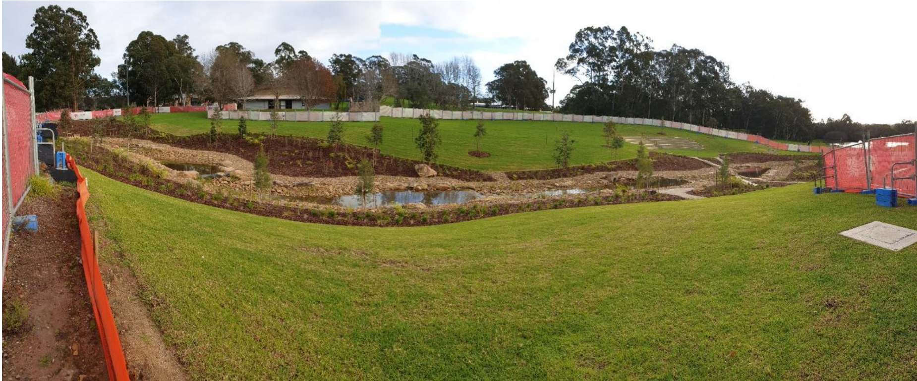
Photo 1 – Landscape works were completed at the creek area and sediment fence was installed along the construction site perimeter. The sediment basin was moved to the right upgradient of the creek. Water in the creek was clear. There was no sign of sediment laden water coming out from the site.
