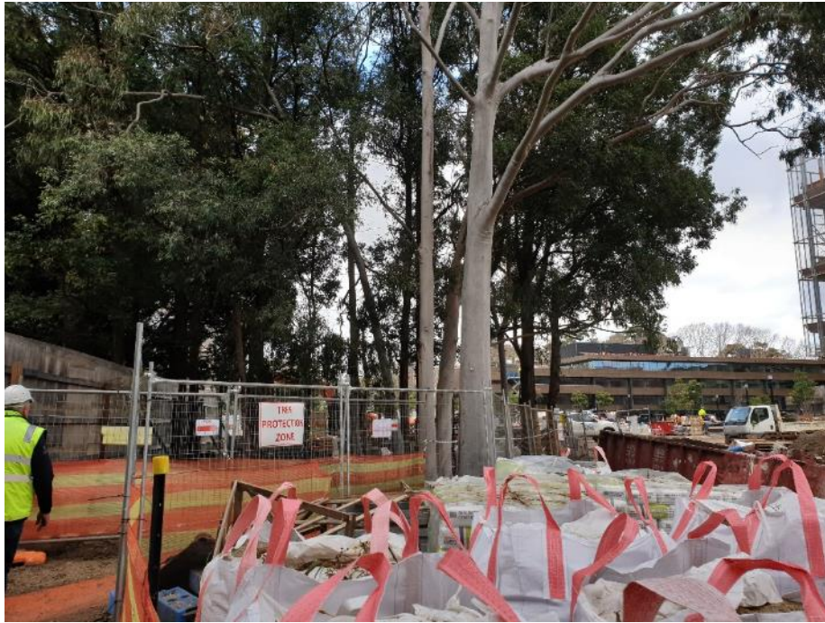
Photo 12 – Tree protection zone were fenced off with signage installed.
