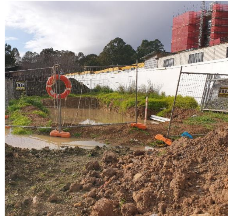
Photo 2 – Sediment basin was relocated and resized. Sediment fence was installed along the perimeter prior to the grass area to the creek. It was also noted that the site detention tank was in operation to accept the stormwater coming from the central courtyard stormwater drains.
