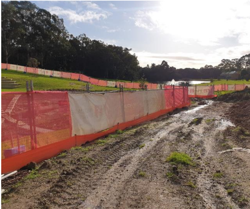
Photo 2 – Sediment basin was relocated and resized. Sediment fence was installed along the perimeter prior to the grass area to the creek. It was also noted that the site detention tank was in operation to accept the stormwater coming from the central courtyard stormwater drains.
