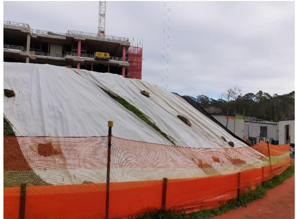
Photo 5 – Stockpile was covered, and sediment fence was installed around it.
