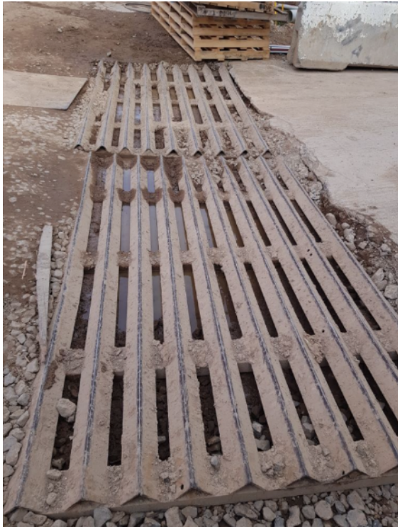
Photo 10 – Rumble grid cleaned after rain event on the day of the audit, photo provided by the contractor.
