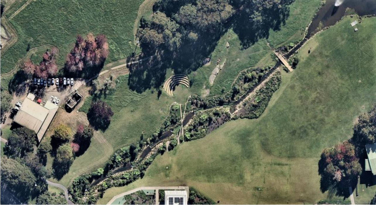
Image 6: An aerial photo indicating the re-constructed Mars Creek Reach 3 in 2022
