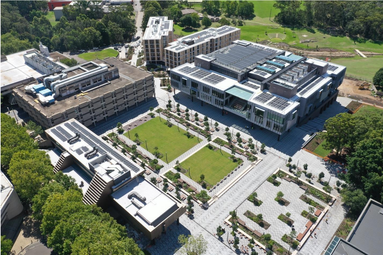
Image 2: MUCCP Central Courtyard Precinct
