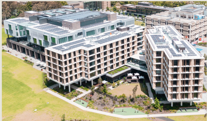
Central Courtyard Precinct rooftop solar Image credit: Joanne Stephan
