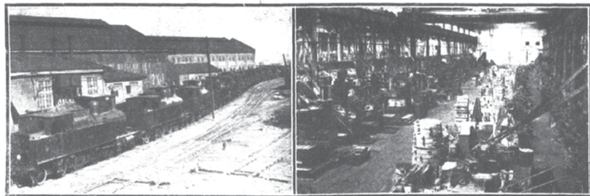
The picture on the left shows a long line of engines outside the Eveleigh sheds. On the right is one of the workshops, absolutely idle.—(Mirror Photos.)
