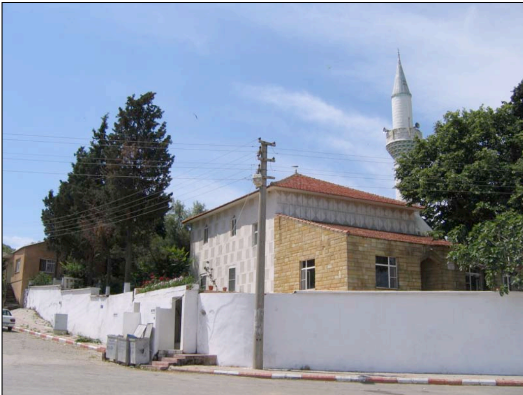
AC 6.II.Ag.6 Gazi Süleyman Pasha Memorial Mosque at Bolayır – the original mosque was heavily damaged by naval gun fire from HMS Agamemnon prior to the Allied landings in 1915. (Photo. SL 2010)
