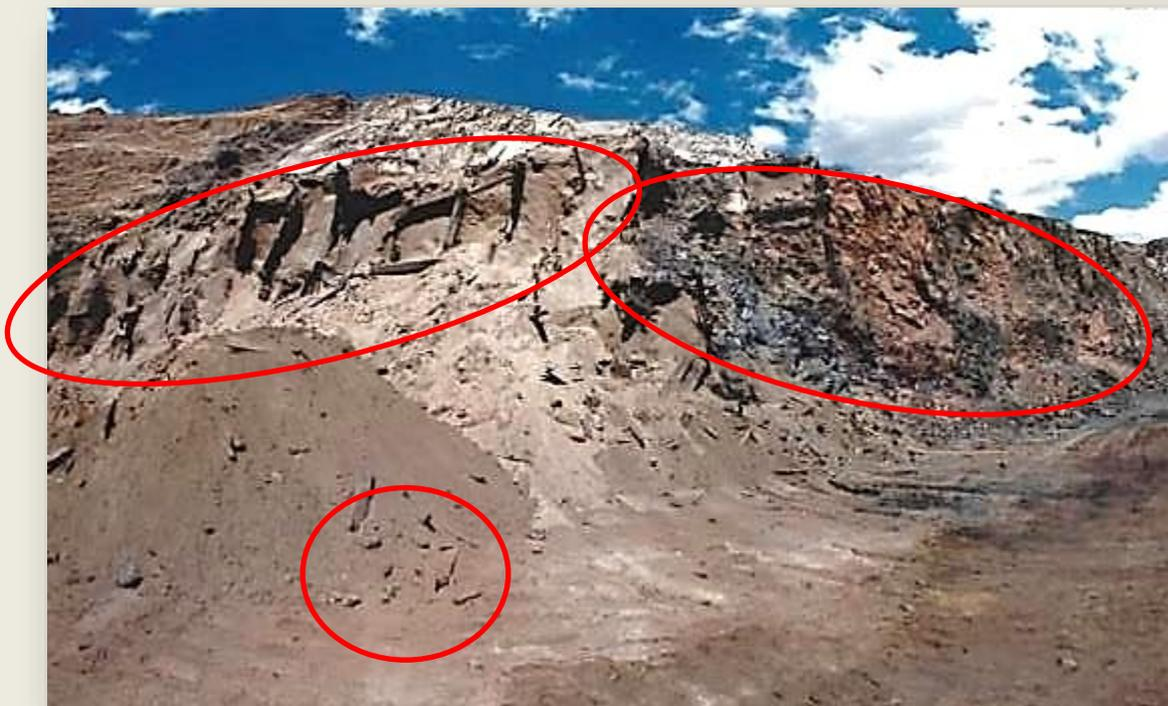
*Oregon square-set timbering* clearly visible, exposed in the Kintore Open Cut mine at Broken Hill. The open cut pit encompassed the original Kintore shaft and underground mine. The stopes had been backfilled with tailings from the mill. Photo: David Edgecombe.
