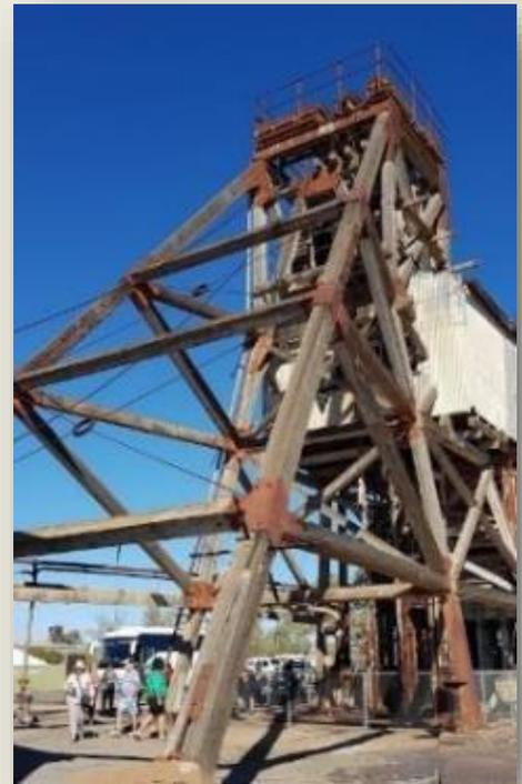
Oregon timber used in the head frame erected over the Browne Shaft at Broken Hill in the 1890s, is still in exceptionally good condition.
