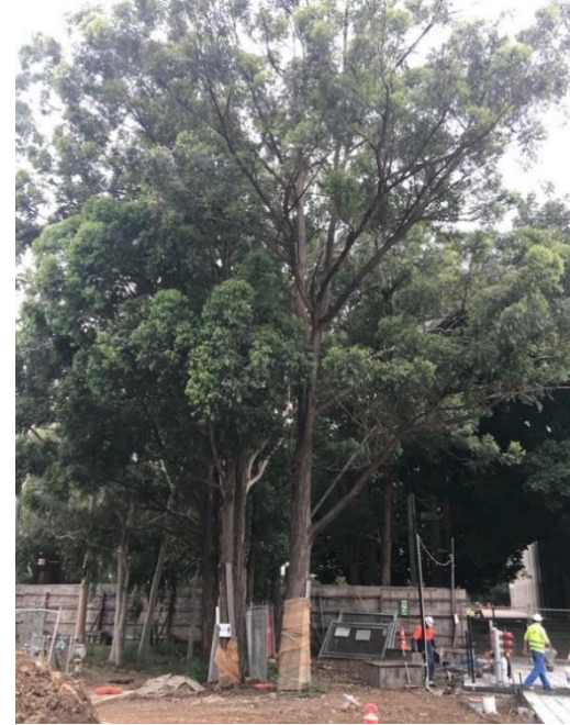
Photo 4 – Tree protection installed around the protected trees.
