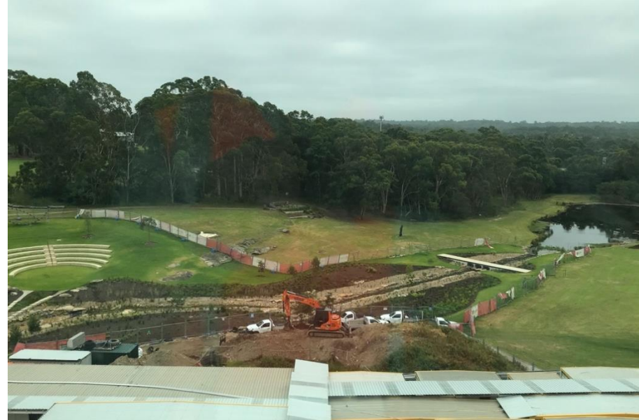
Photo 6 – Stabilised stockpile behind site sheds with silt fence installed along the perimeter.
